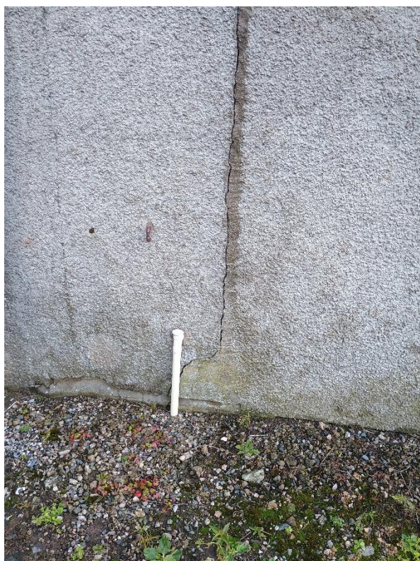
Figure A4 & A5. Vertical crack on extension gable with signs of defective historic repair
