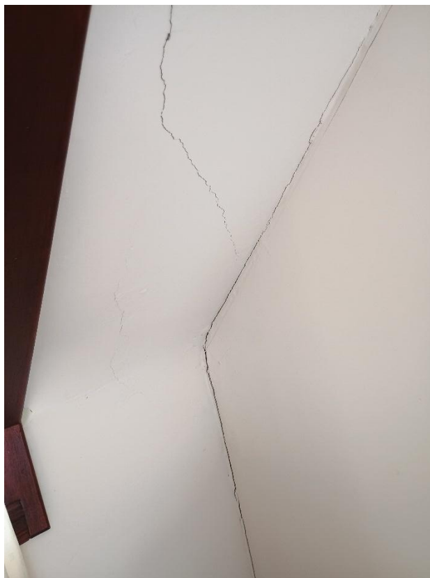
Figure A7. Internal cracking at the corner of the first floor bedroom correlation with the external crack as indicated in Figure A1.
