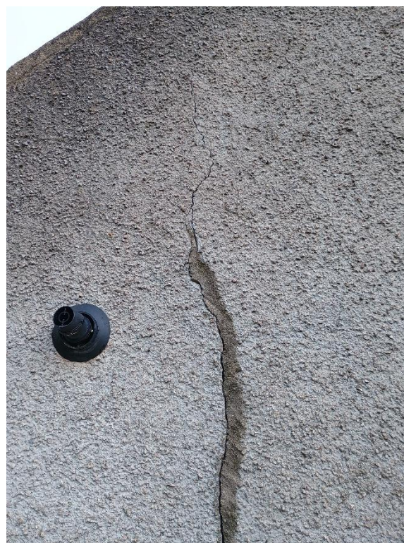
Figure A4 & A5. Vertical crack on extension gable with signs of defective historic repair
