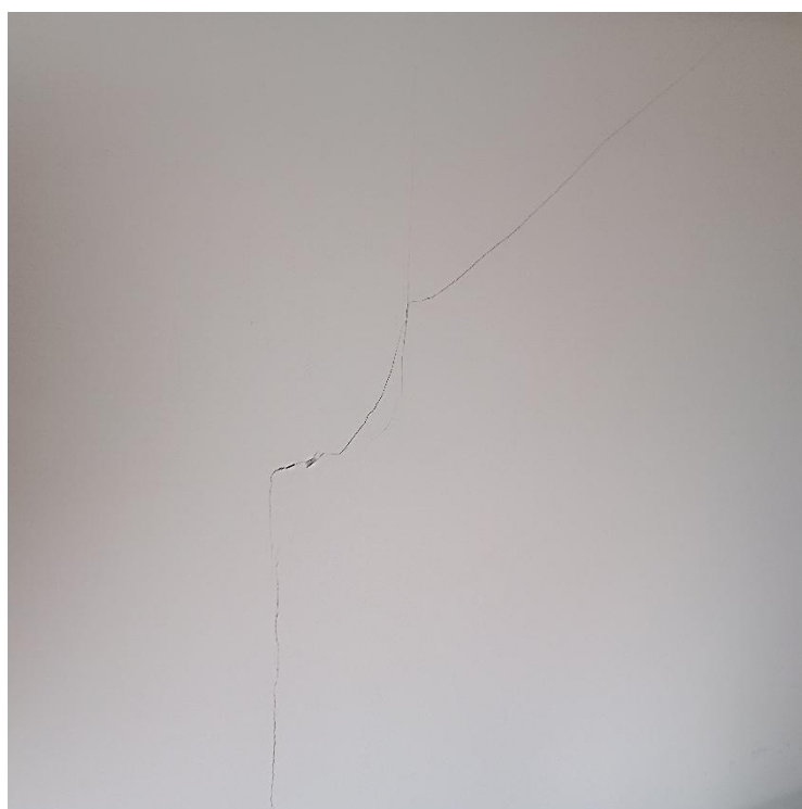
Figure A9. Hairline to fine cracking as typically observed on internal wall finishes
