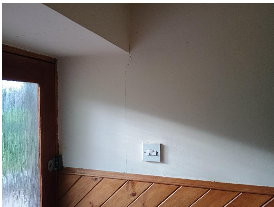
Figure A8. Internal cracking observed at the extension door
