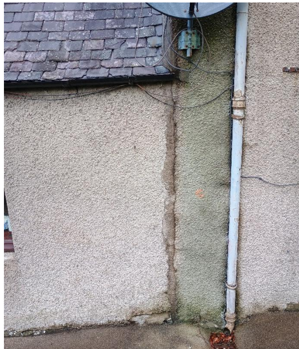
Figure A2. Cracking at joint between extension and original building
