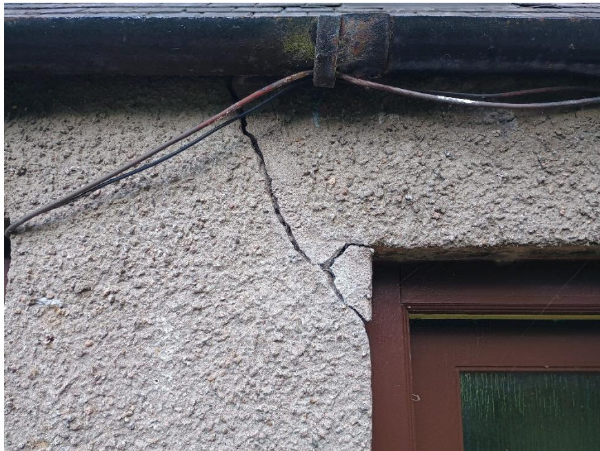
Figure A6. Cracking at the extension door
