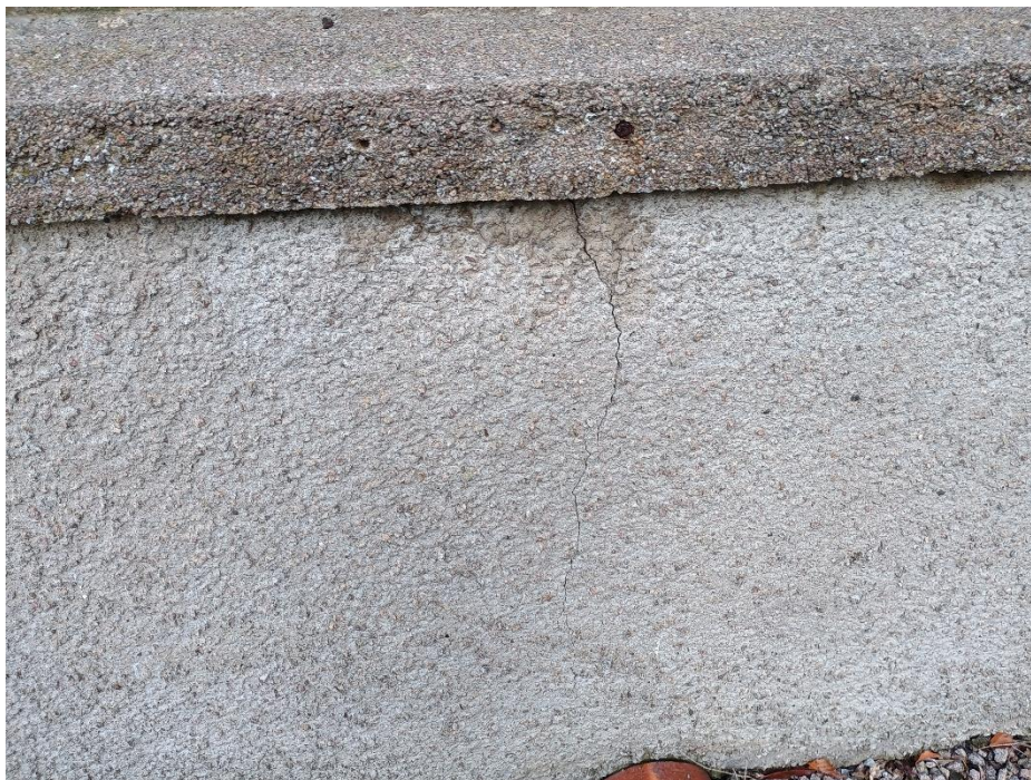
Figure A3. Hairline to fine cracking below the sill of the window of the kitchen at the extension kitchen
