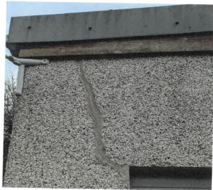
Figure 2 Filled crack above the left-hand garage door.
