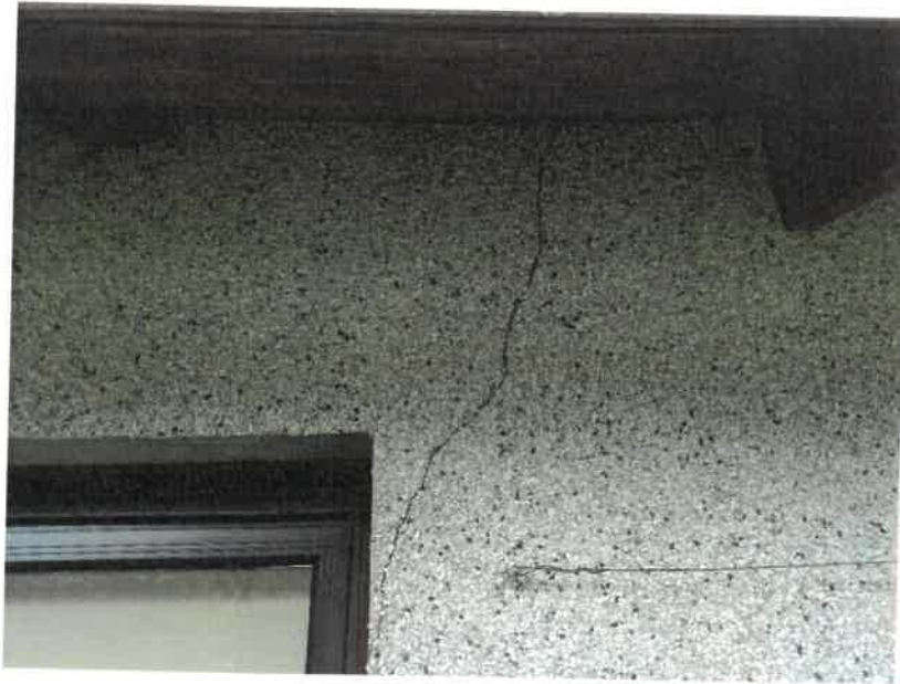
Figure 3 Crack to rear elevation. The crack fades to a hairline width below the area shown.
