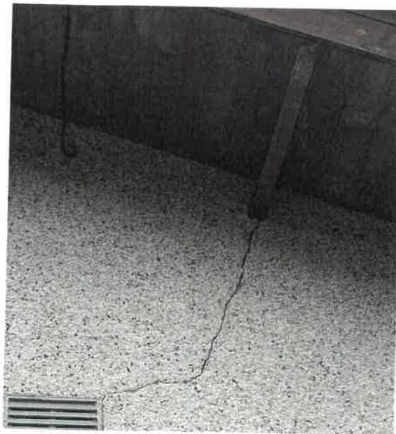
Figure 4 Diagonal crack to right gable wall
