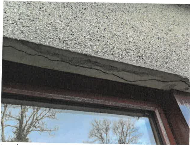
Figure 5 Cracking to the render on the underside of the window opening on the right gable wall. A further hairline horizontal crack is present about 200mm above the opening although not clearly visible in the image.
