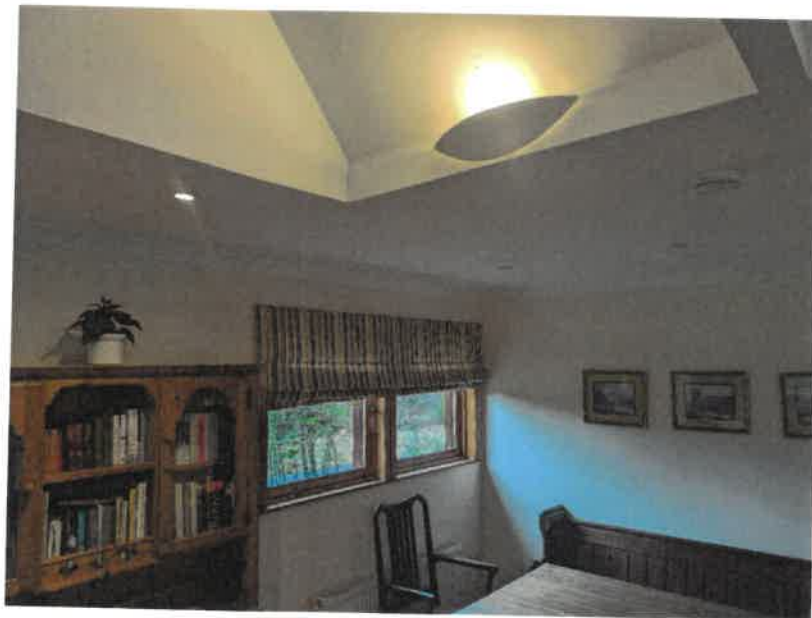
Figure 6 Typical internal view showing painted plasterboard finishes with no cracking. The left side of the image is the right gable wall of the property.
