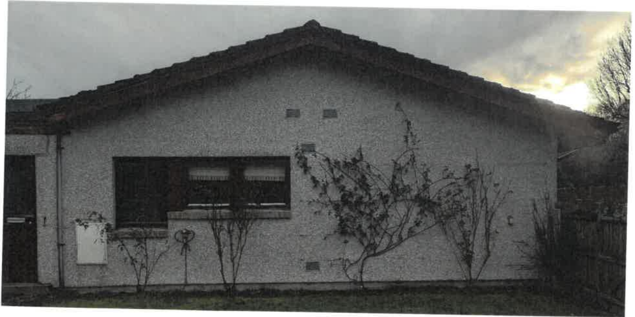
Figure 1 General view of the right gable wall. A filled crack above the doorway is visible and a diagonal crack running from the top-right of a vent to the roof line.
