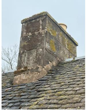
Chimney stacks require raking out of joints in sandstone and repointing using lime mortar mix.
