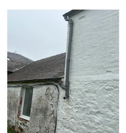
Roof has been re slated at some point and has a non breathable felt to underside unfortunately it has been re slated with wrong type of nail, nails are to short and to thin.
