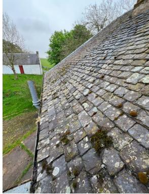
Slates turned on main roof to expose nail heads which were found to be in a good condition, considering age of roof.
