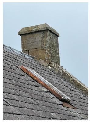
Chimney stacks and skew stones require to be raked out at joints and repointed using a lime mortar mix.
