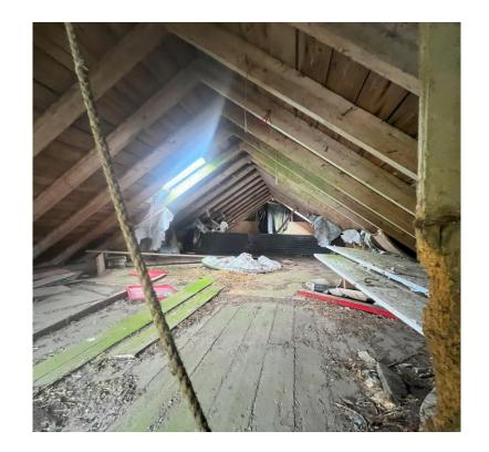
This roof is attached to Roof 9, this lean to slated roof has failed due to being slated using wrong size of slate,
