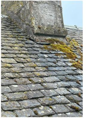
Roof 2 is slated with a Welsh slate; this roof is part of an extension added later to property. Nail heads were found in a fair condition.
